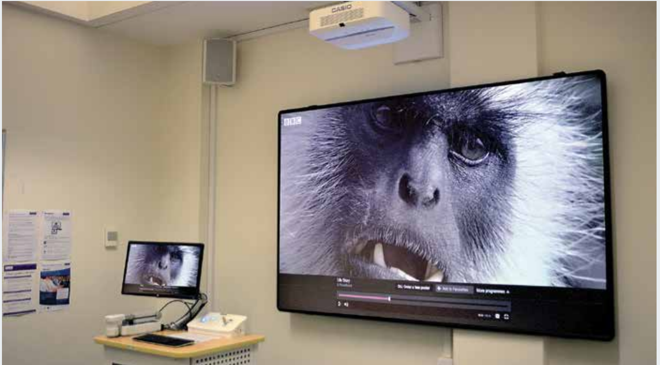
Ultra Short Throw projection solved visibility problems caused by undersized flat panels for University of Manchester's multi-purpose study rooms
